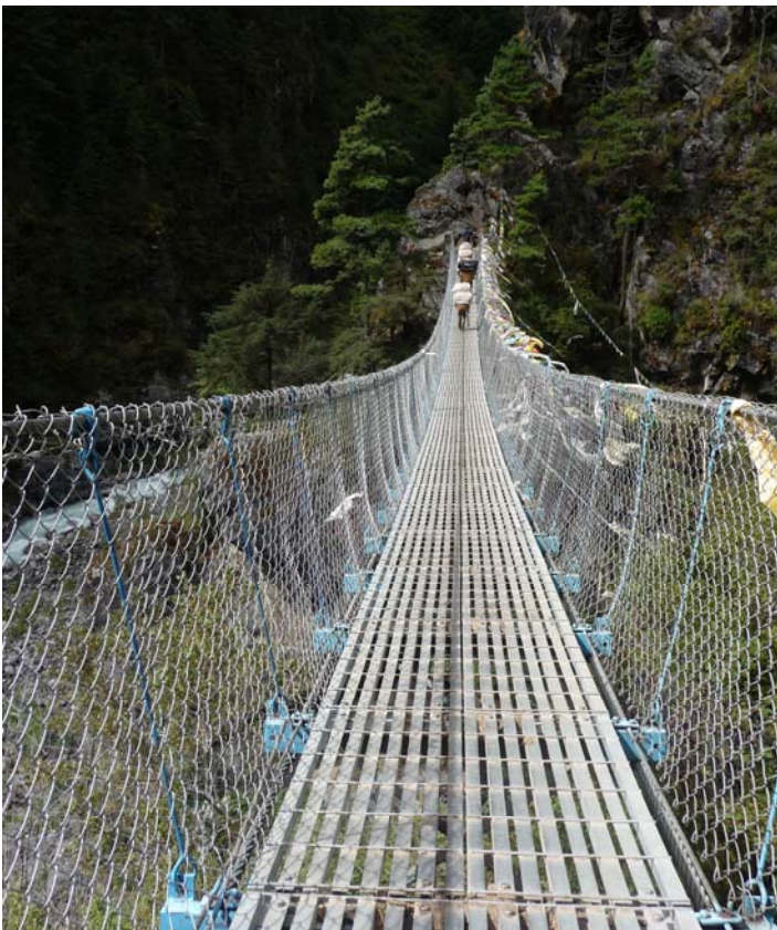
Don't look down: Typical Himalayan bridge.
