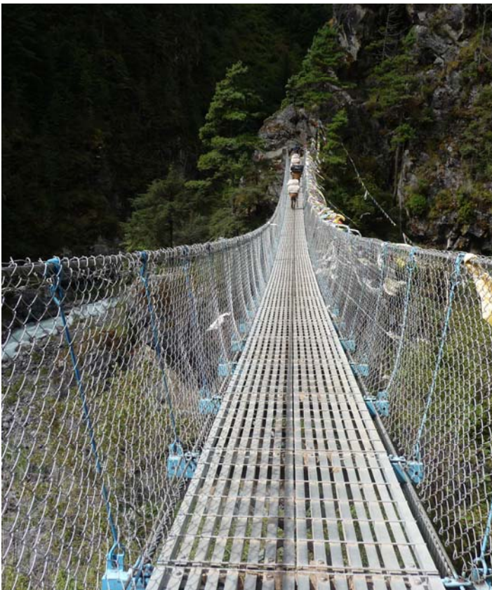
Don't look down: Typical Himalayan bridge.
